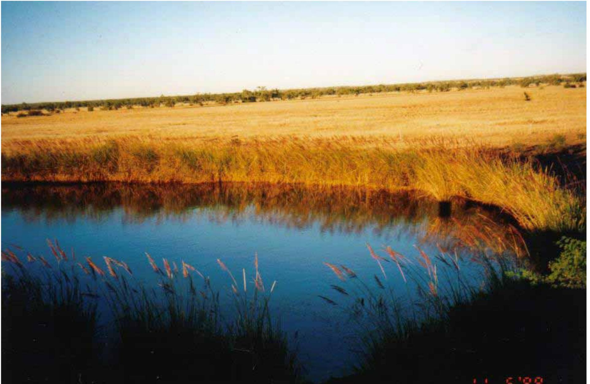
**Inside wall of a large farm dam in northern Australia to control wave erosion**
